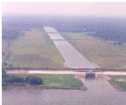
Freshwater diversion canal at Davis Pond.
