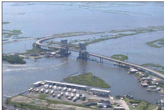
LA 1 Bridge in Leeville, Louisiana
